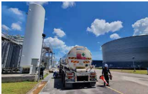
Maintenance of water reservoir at workers' camp at PIC
